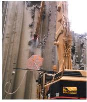
The basic nozzle installation aims high pressure water jets CONTINU-OUSLY to the working zone of crusher, i.e. practically between crusher's jaws, when the water consumption is kept app. at 10 – 15 l/min.
